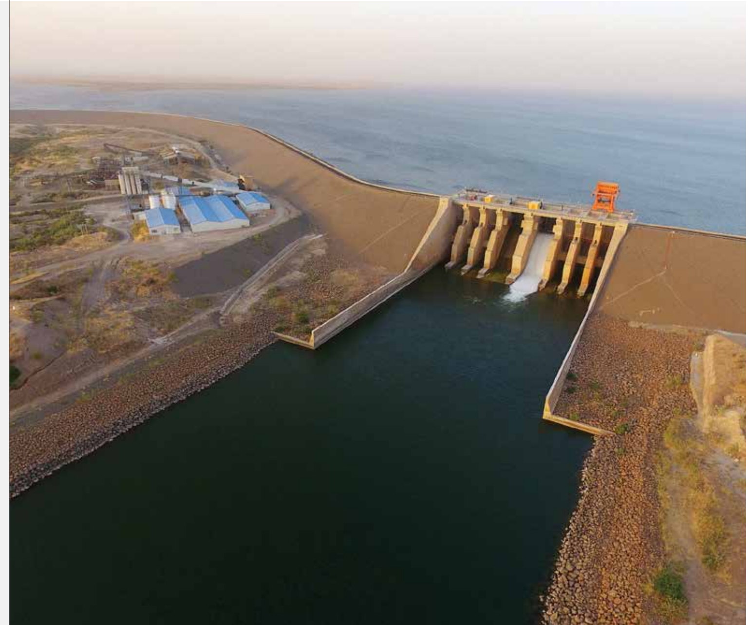
Upper Atbara Dam - Sudan
